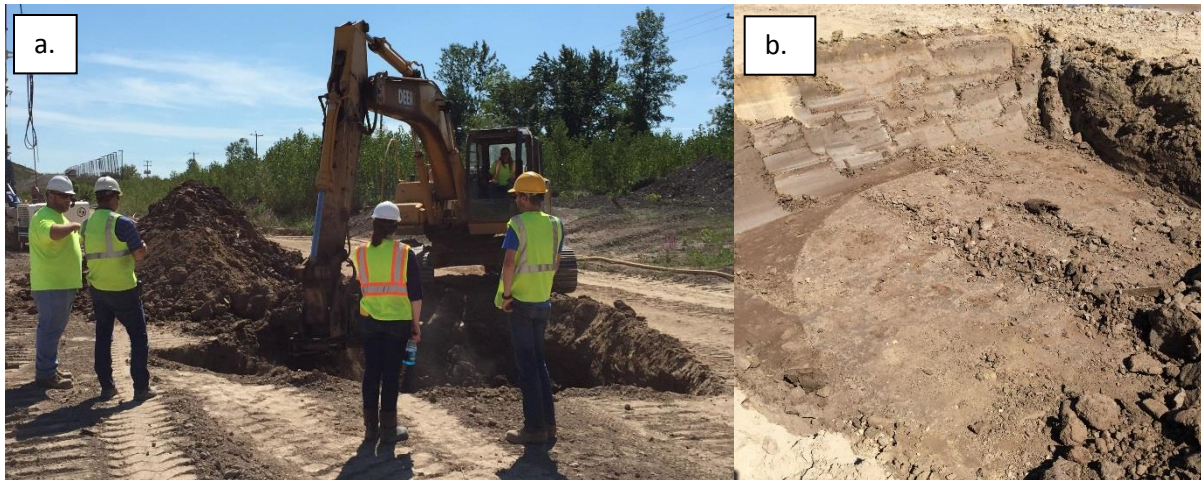
Figure 6. Column Excavation (a) and exposed column (b) in Stage 6
