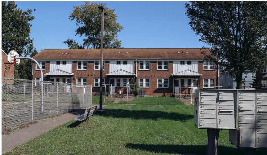
Saratoga Sites, a public housing complex in Cohoes, N.Y. , was recently closed due to community concerns over air pollution from the nearby Norlite hazardous waste-burning plant .
