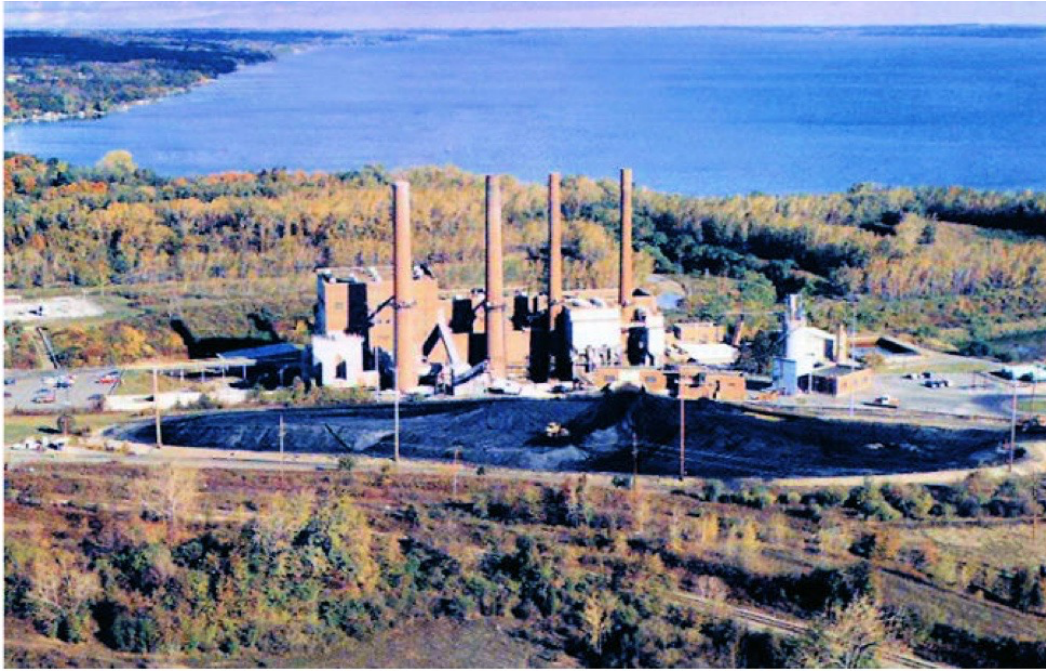
The Greenidge Generation power plant in Dresden restarted in March 2017.
