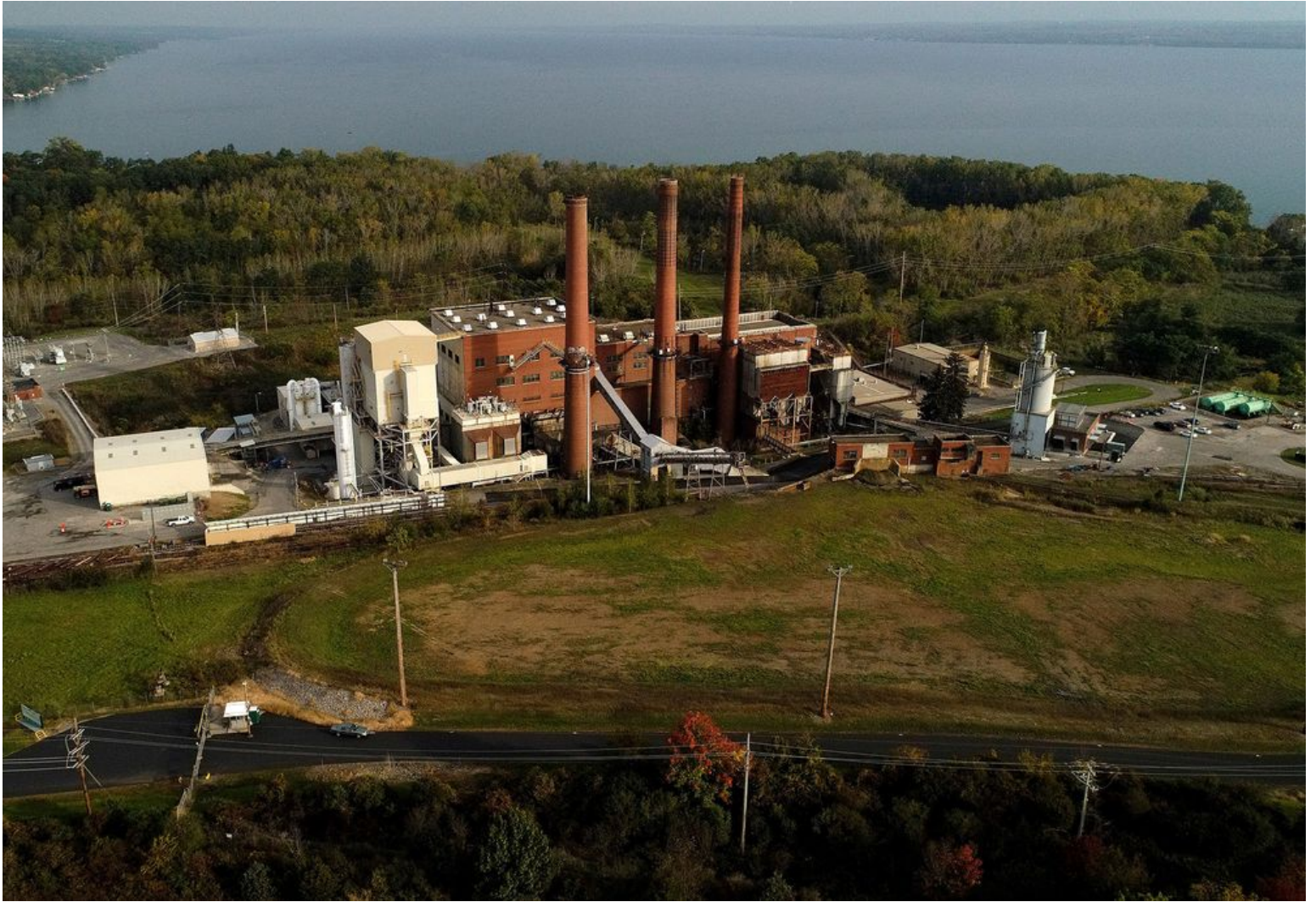
The Greenidge Generation power plant on the banks of Seneca Lake, in Dresden, New York. Source: Shutterstock
