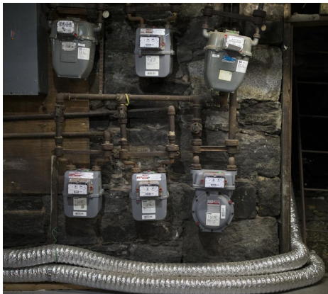
BROOKLYN, NEW YORK - JULY 4: Six meters placed by National Grid measure natural gas consumption in a ... [+] GETTY IMAGES
