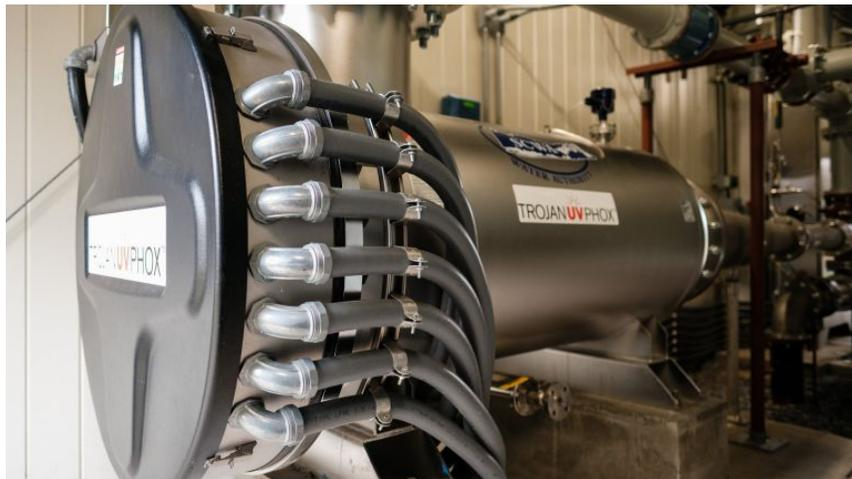
The Suffolk County Water Authority's Advanced Oxidation Process treatment system, designed to remove the contaminant 1,4-dioxane from groundwater, at the SCWA Commercial Boulevard pump station in Central Islip in December 2018. Photo Credit: Barry Sloan
